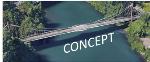
**Project Scope:** To reconstruct an all-new pedestrian bridge over the Umatilla River to replace the bridge that was damaged by the 2019 and 2020 floods. Includes raising the bridge by approximately 5' and extending it by approximately 120' in length. Also includes replacing the 18" waterline that was damaged with two 24" waterlines.
