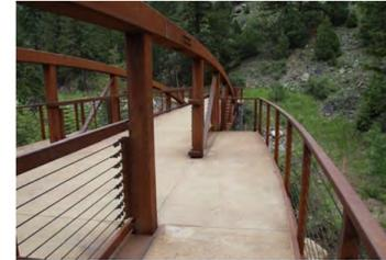
**Project Scope:** To reconstruct an all-new pedestrian bridge over the Umatilla River to replace the bridge that was damaged by the 2019 and 2020 floods. Includes raising the bridge by approximately 5' and extending it by approximately 120' in length. Also includes replacing the 18" waterline that was damaged .
