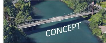
**Project Scope:** To reconstruct an all-new pedestrian bridge over the Umatilla River to replace the bridge that was damaged by the 2019 and 2020 floods. Includes raising the bridge by approximately 5' and extending it by approximately 120' in length. Also includes replacing the 18" waterline that was damaged.
